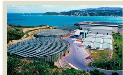
Clearwater at Moa Point Treatment Plant. Photo courtesy of Neil Price, Wellington City Council.
