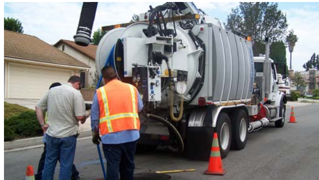
Photo 4: The line cleaning crew at work as a member of the analysis team looks on
