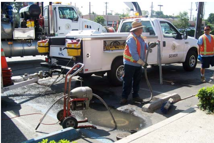
Photo 2: The lateral rodding crew responding to a commercial lateral blockage that threatened to enter a public drain.
