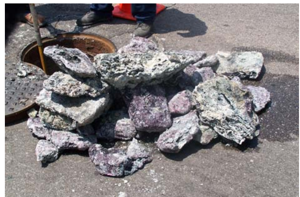
Photo 8: Grease "rocks" removed from Magnolia sewer line
