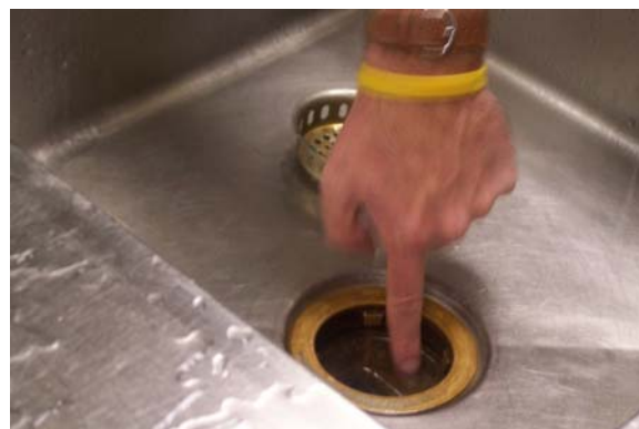
Photo 7: The Source Control Inspector checking a drain for grease build-up during the Morningside inspection.
