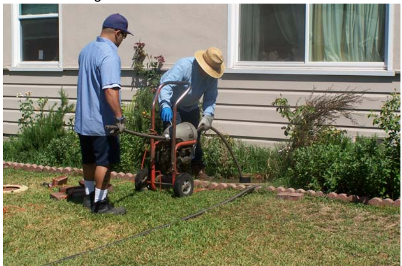
Photo 11: The lateral crew operating the rodding machine
