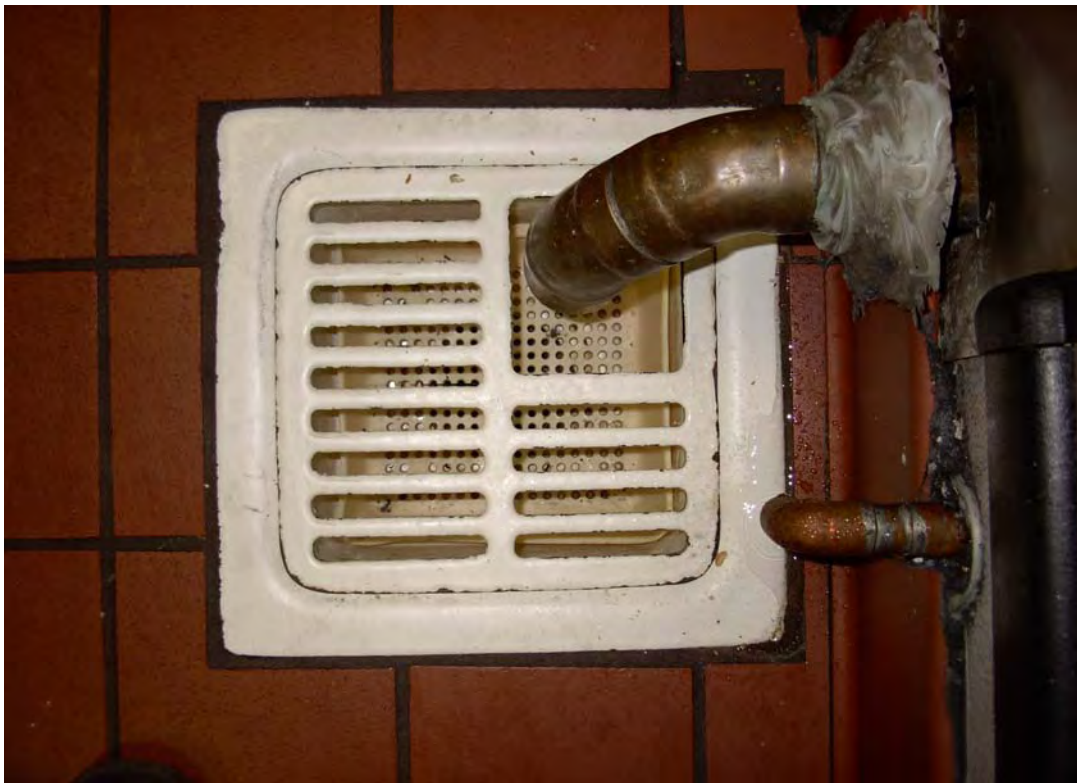
FIGURE 6-3 Floor Sink with a Drain Screen
