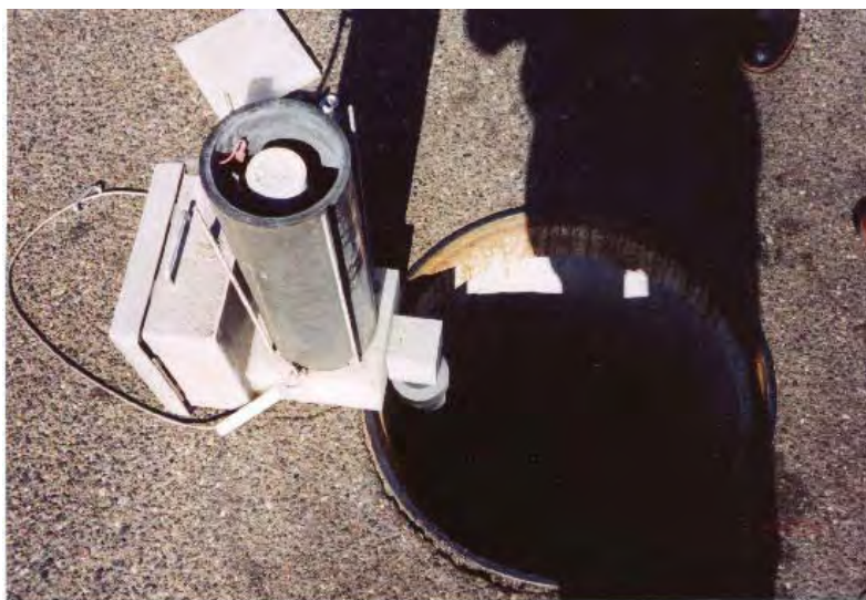
3. Top of feeder removed to refill with additive.
