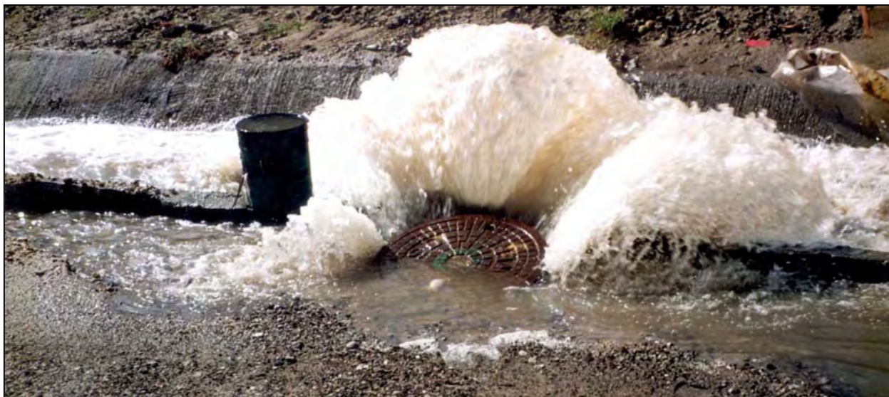
FIGURE 1-1 Sewer overflow (Courtesy of County Sanitation Districts of Los Angeles County)
