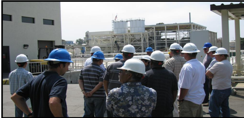
Heat Dryers at Encina Wastewater Authority
