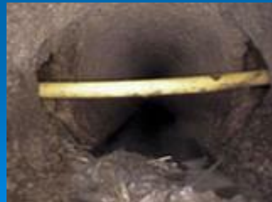
Gas Line Bored Trough
