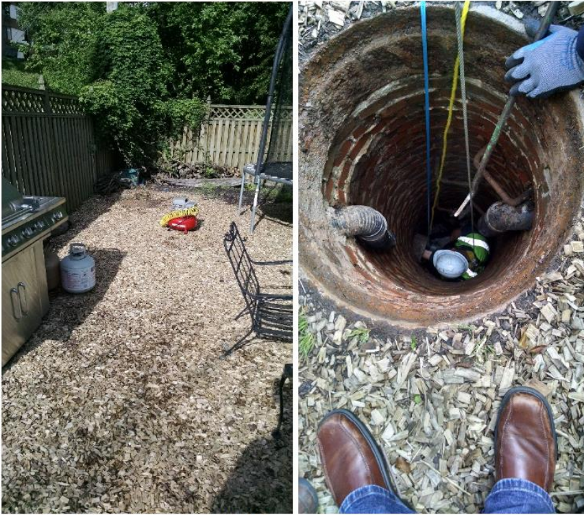
Figure 3. Installation at the Downstream Manhole
