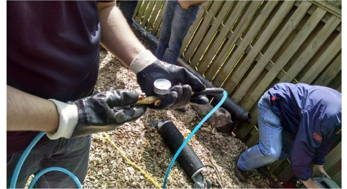
Figure 4. Manual Plug Inflation
