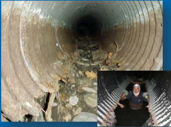
Deteriorated Bottoms
