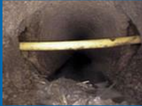
Bored Gas Lines
