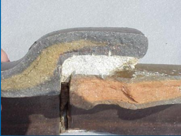
Top of Pipe Joint Grouted
